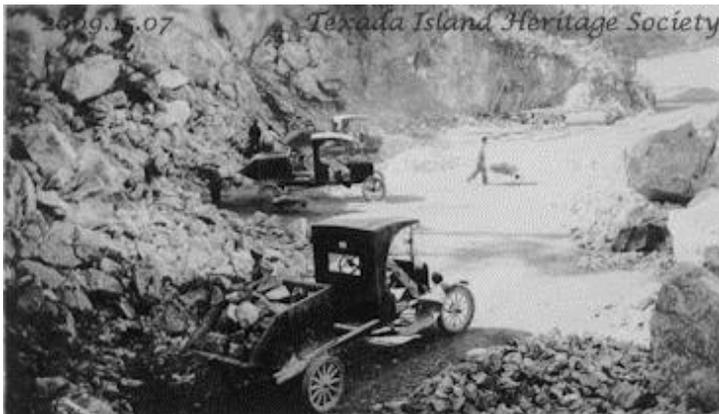
Lime rock was "shot out" of the cliffs, drilled, then broken by hand hammer. The hundred-pound "man-sized rock" was muscled onto the small 1924 Model-T Ford dump truck by the "B&L" (Breaker and Loader) crew. It is reported that Big Joe Little could easily lift and carry even larger pieces.
